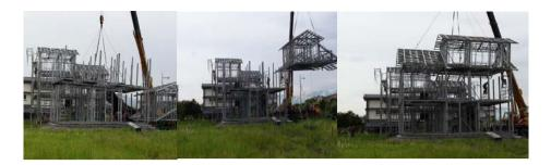
Figure 3-8 Illustration of Building the Steel Framework of the AG Innovative Composite Structure
