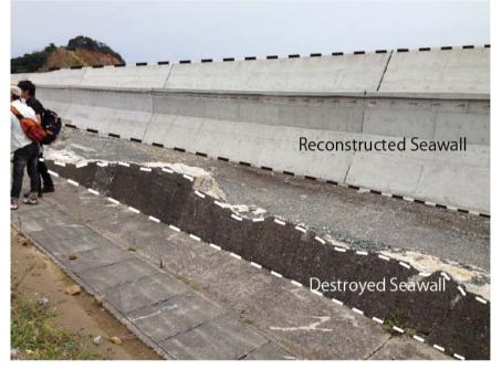
Photo 1. Seawall reconstruction on the same site is easy way
